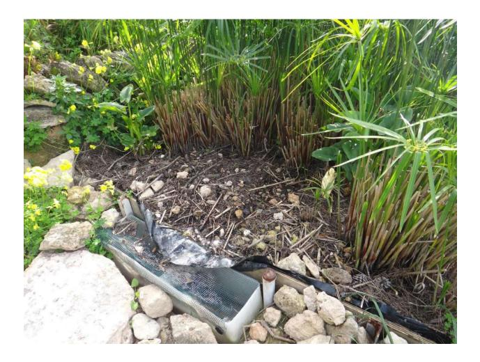
The filtered water enters in the 'Tipper box' (an apparatus used for the distribution of grey water to the vegetable gardens)
