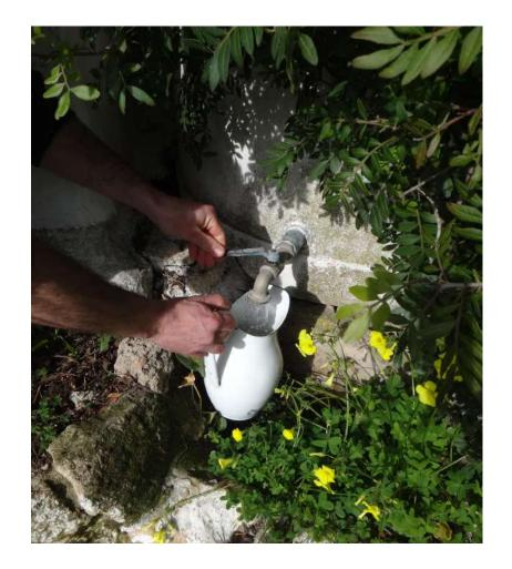
The rain water enters the tank from a channel around the toilet roof, which is made from an old satellite dish
